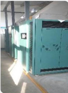
BEFORE: Previously, condensate water from the pure water system was discharged directly, leading to unnecessary waste.
